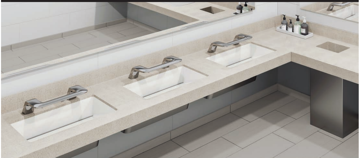
Bradley’s washing bar sinks and hardware in a commercial washroom today.
